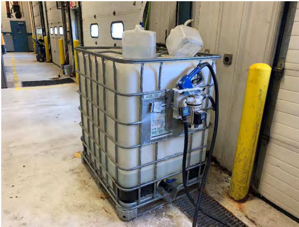
Photograph Tote of diesel fuel emission control additive in maintenance bay inside No 7 Operations Building.
