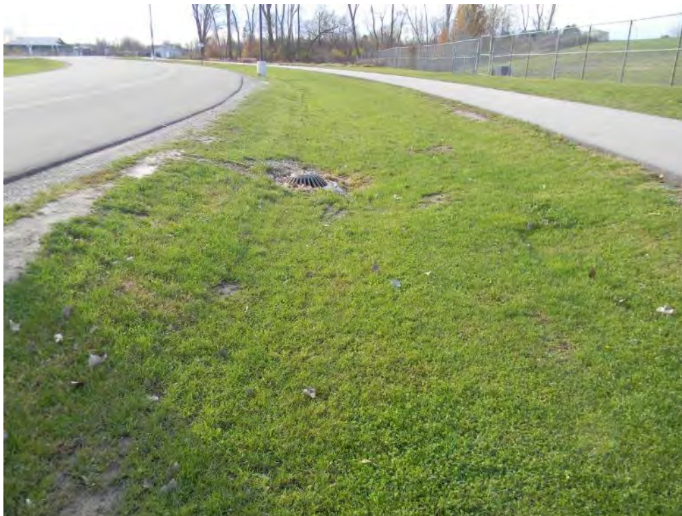
Drainage swale with catch basin along east side of access drive to the north of Beagle Middle School.
