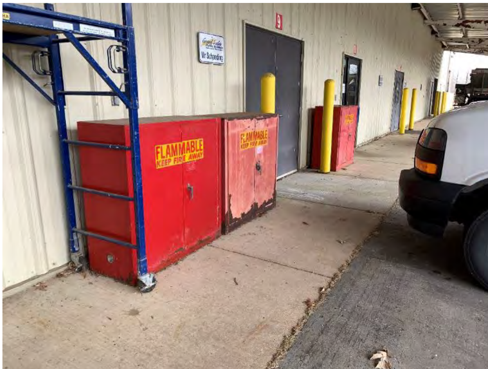
Flammable liquid storage cabinet beneath canopy in storage area along south side Operations Building.
