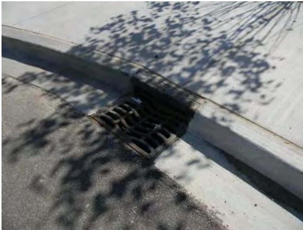
New pavement and catch basin in Holbrook Elementary parking lot.
