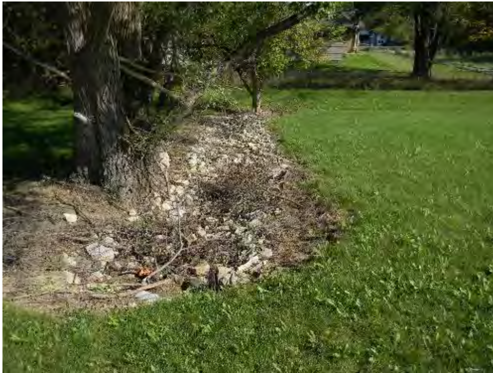
Drainage swale with rocks to detention basin at Wacousta Elementary.
