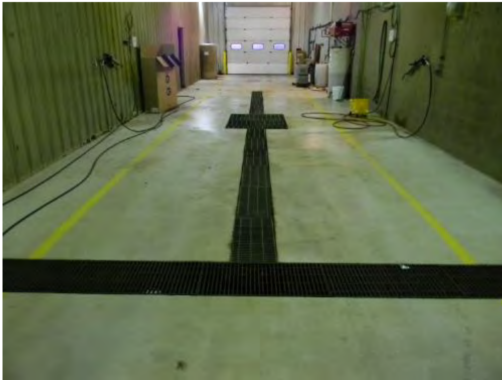
Photograph No 7 View of vehicle wash bay inside Operations Building.
